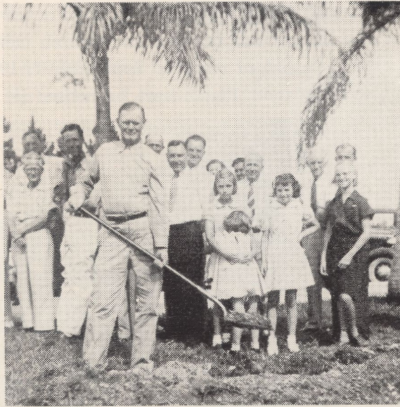
GROUNDBREAKING OF NEW CHURCH
