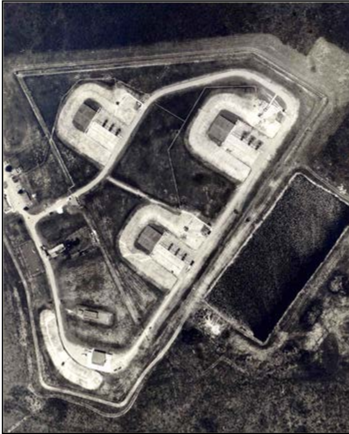
Figure 17-8. Nike Missile Base HM-69, aerial view of launch area
