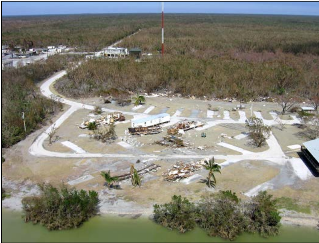
Figure 16-4. Flamingo housing area following Hurricane Wilma, 2005
