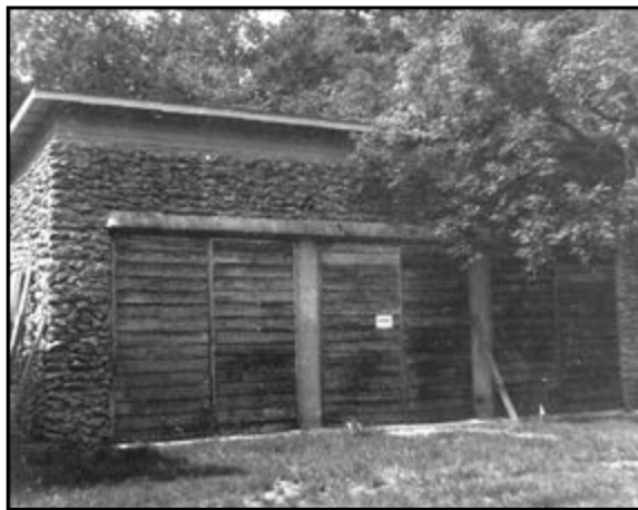
Figure 17-7. Civilian Conservation Corps-built garage at Royal Palm, 1950 photo
